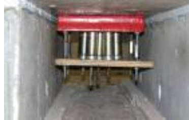
(c) Base of footing
