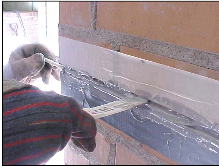
Fig. 3.3.4f Embedding of GFRP bar into the joint
