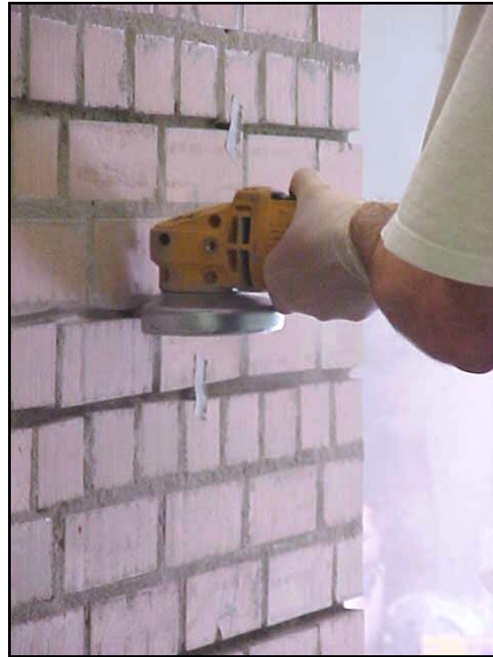
Fig. 3.3.4b Grooving along the mortar joint
