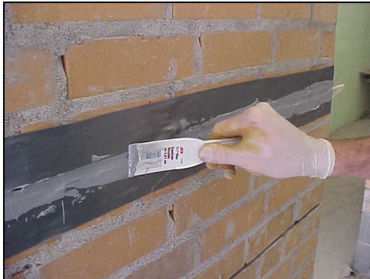
Fig. 3.3.4g Final retooling of the joint
