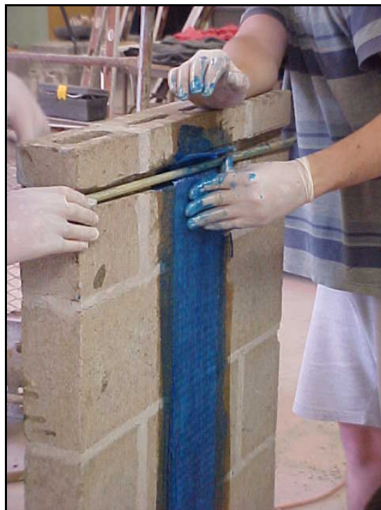
Fig. 2.3.3k Installation of GFRP rod as anchorage
