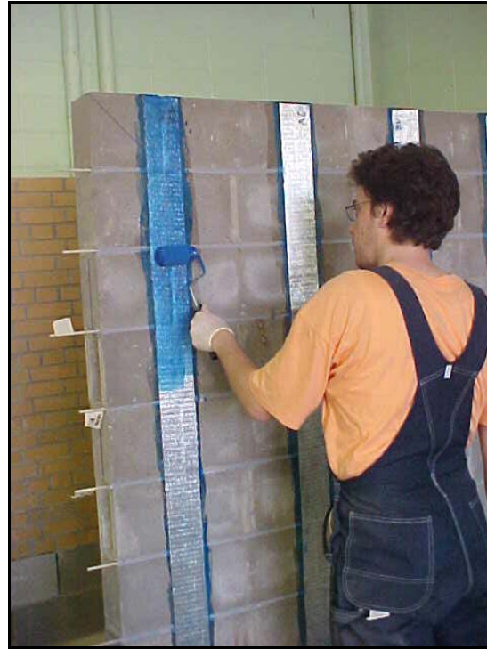
Fig. 3.3.4n 2 nd coat of saturant
