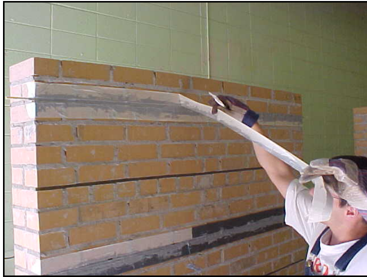
Fig. 3.3.4h Removal of the masking tape
