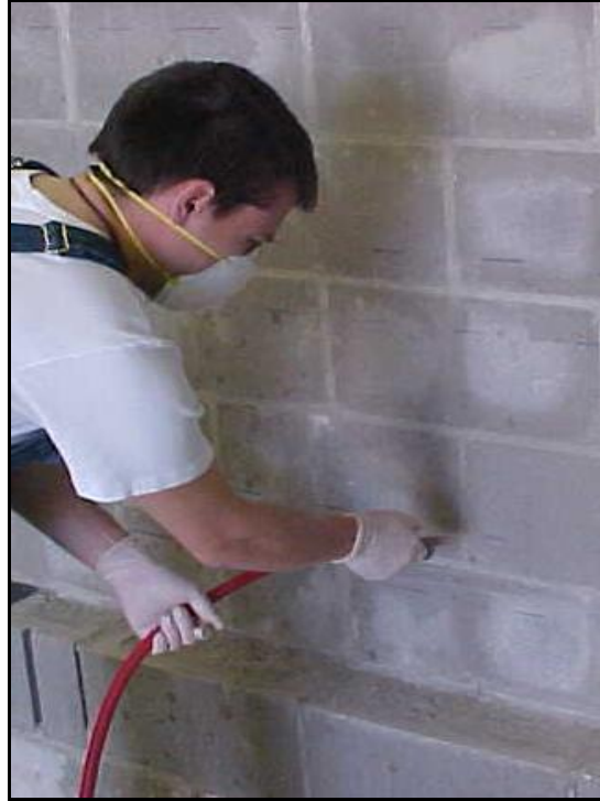
Fig. 2.3.3b Removing of dust and any loose particles
