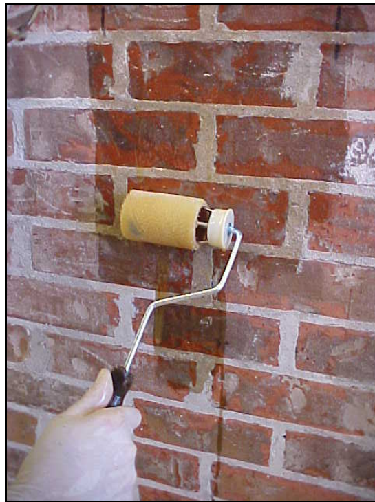
Fig. 2.3.3c Application of primer on clay
