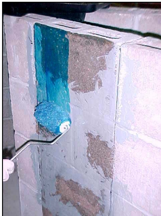
Fig. 2.3.3e First coat of saturant
