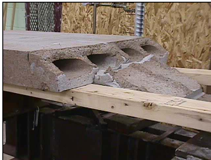
Fig. 2.3.5h* Shear fractures on masonry units
