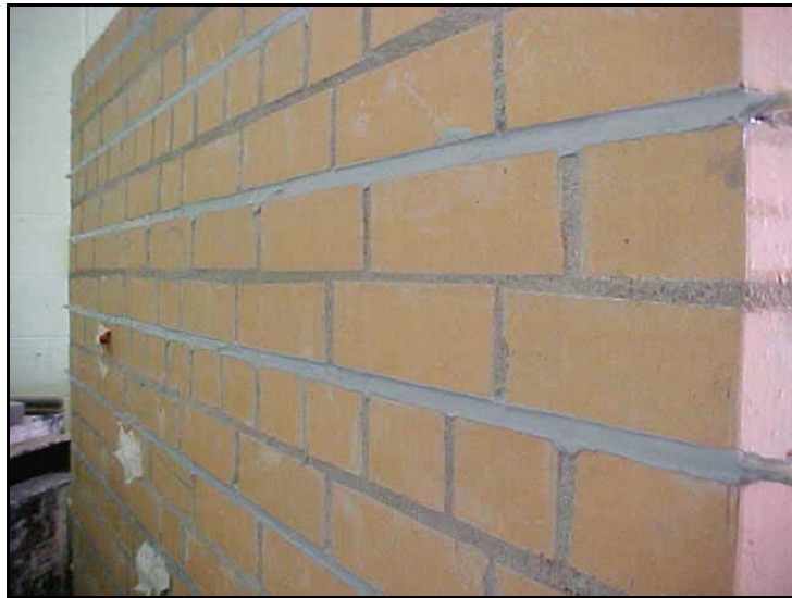
Fig. 3.3.4i Masonry surface after strengthening
