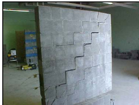
Fig. 3.5.1d Unstrengthened side of the wall after failure
