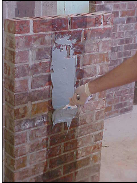
Fig. 2.3.3d Leveling with putty
