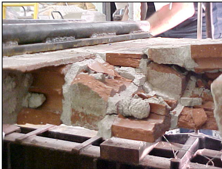
Fig. 2.3.5l Shear failure with separation of masonry elements
