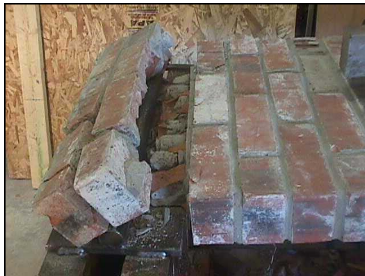
Fig. 2.3.5j*** Shear failure at the edge
