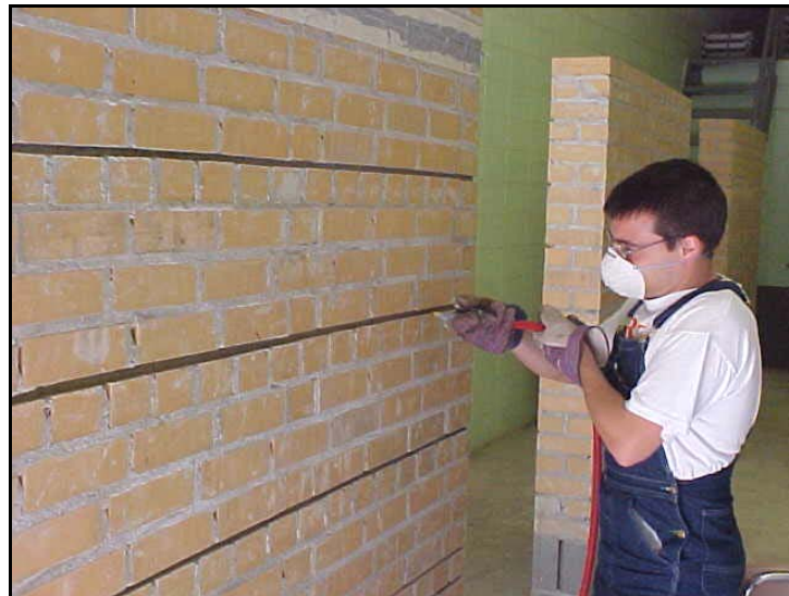
Fig. 3.3.4c Removal of dust by air pressure
