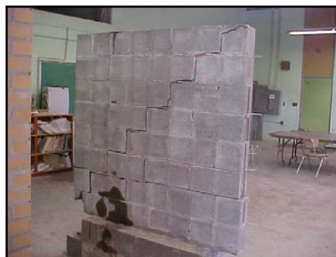
Fig. 3.5.1h Cracked wall after failure
