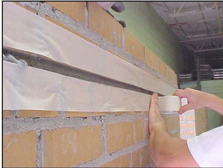
Fig. 3.3.4d Masking of masonry to avoid staining
