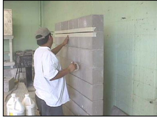
(2) Masking to avoid staining
