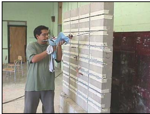
(3) Application of epoxy-based paste
