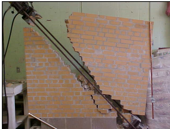
Fig. 3.5.2b Collapse of the unstrengthened wall
