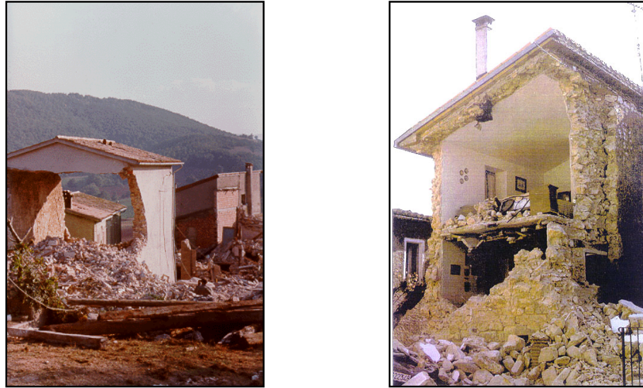
Fig.1.1.1 a-b Out-of-plane collapse of bearing walls Umbria, Italy, 1997
