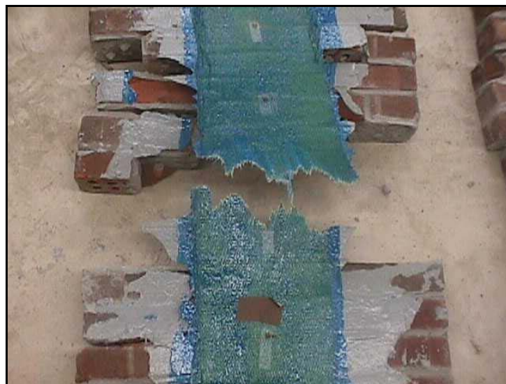
Fig. 2.3.5h*** Rupture of the AFRP laminate
