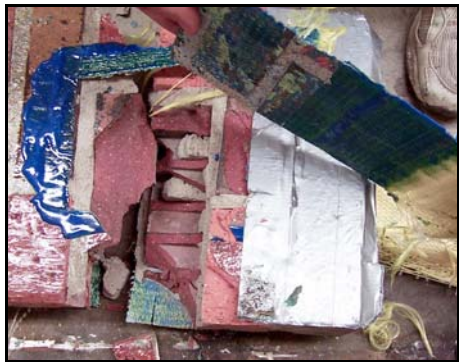
(e) Damage in masonry bricks
