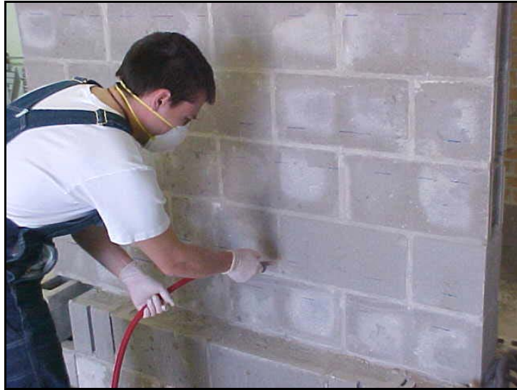
Fig.3.3.4j Removal of any loose parts from the masonry surface
