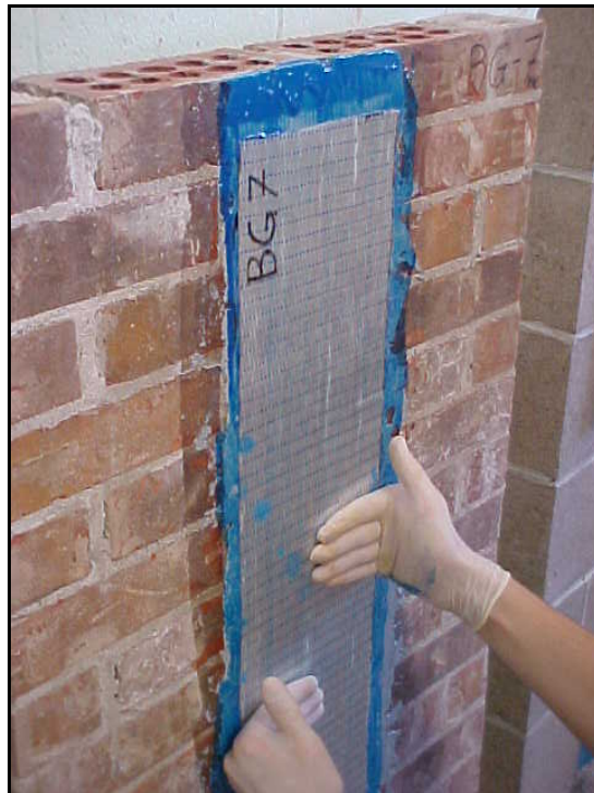
Fig. 2.3.3g Fiber installation
