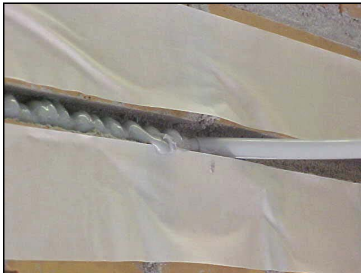
Fig. 3.3.4e Injection of epoxy-based paste into the groove
