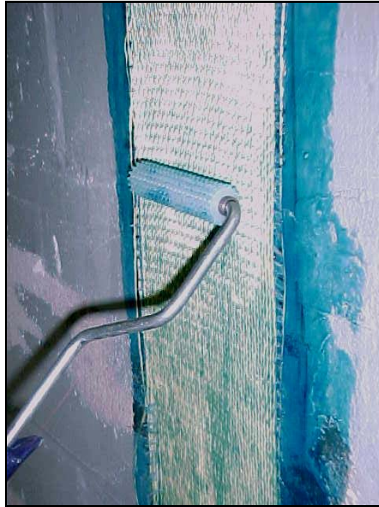
Fig. 2.3.3h Elimination of air bubbles
