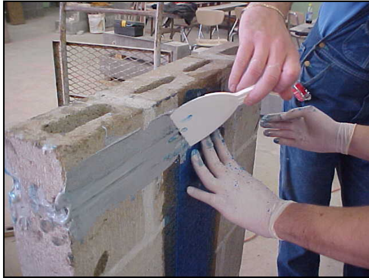
Fig. 2.3.3l Injection of epoxy-based paste into the groove and final retooling
