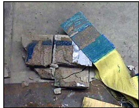
(f) Damage in concrete blocks
