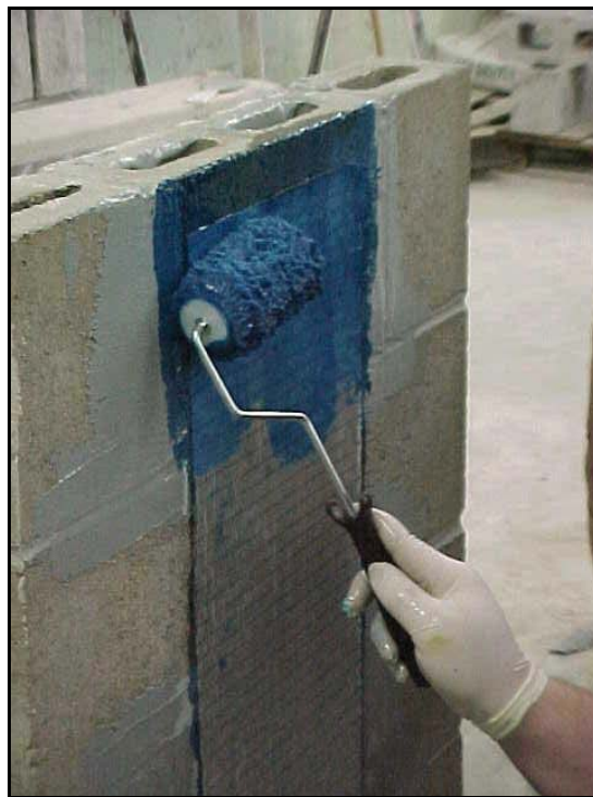
Fig. 2.3.3i Second coat of saturant
