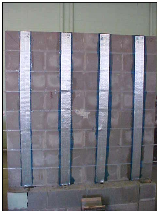
Fig. 3.3.4m Installation of GFRP laminates
