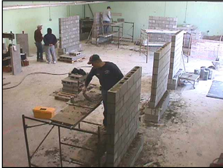
Fig. 3.3.1a Concrete block panels in the testing room
