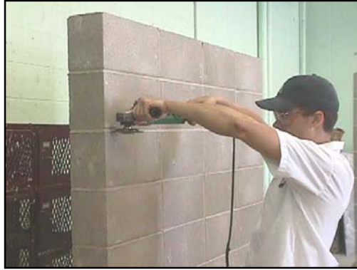
(1) Grinding of joints
