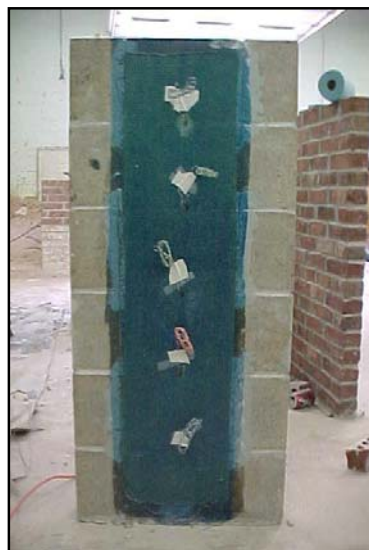
Fig. 2.3.4.2a Placing of strain gages on FRP
